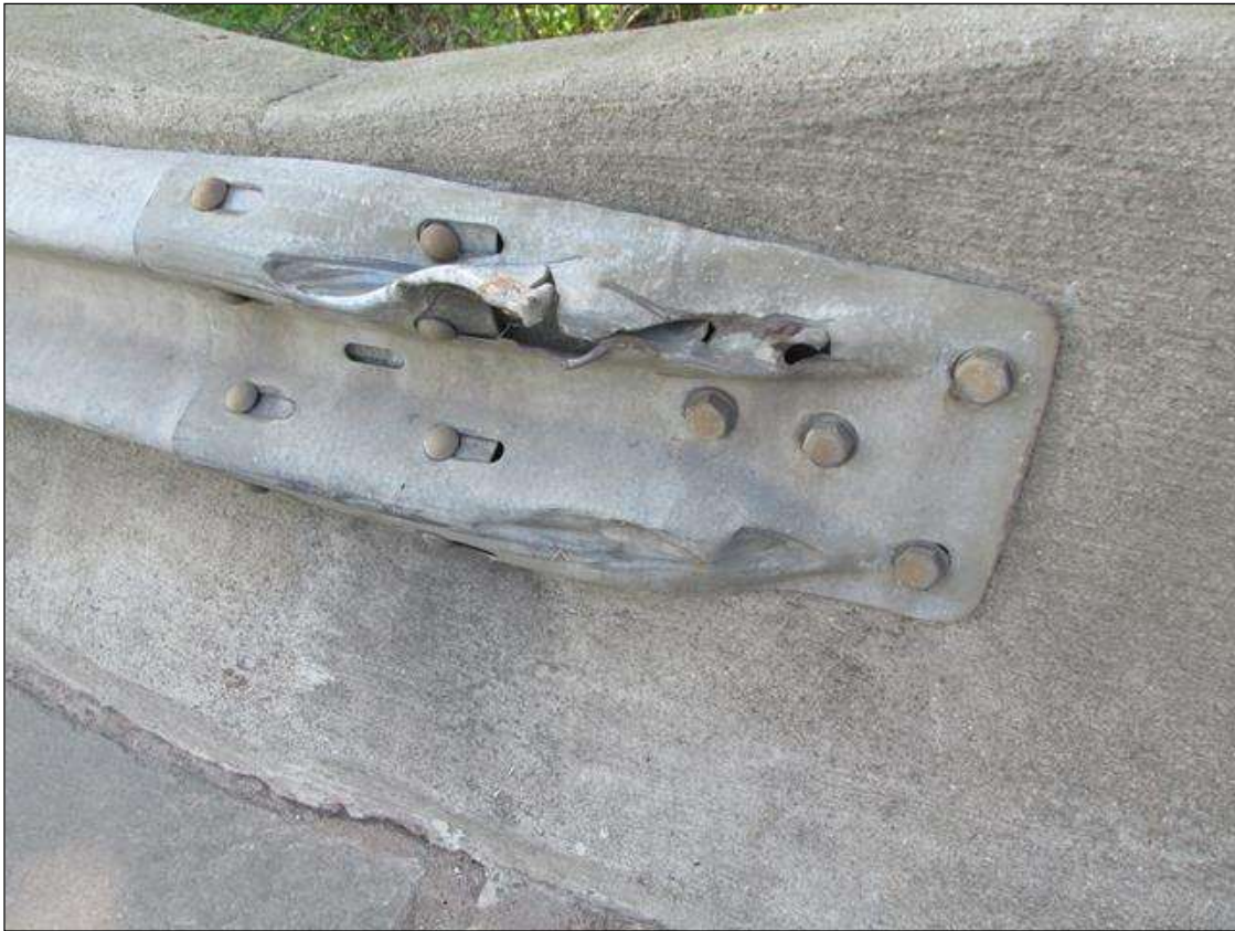
GR CONNECTION DAMAGE, NORTHEAST CORNER. CONNECTION IS NOT LOOSE.
