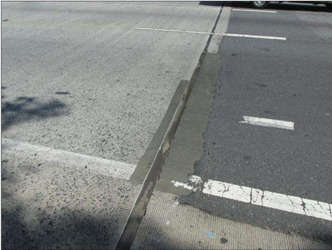
TEMP REPAIR TO DECK AND APPROACH, -L- RT AT NORTH APPROACH, APPROX 10'L X 2'W
