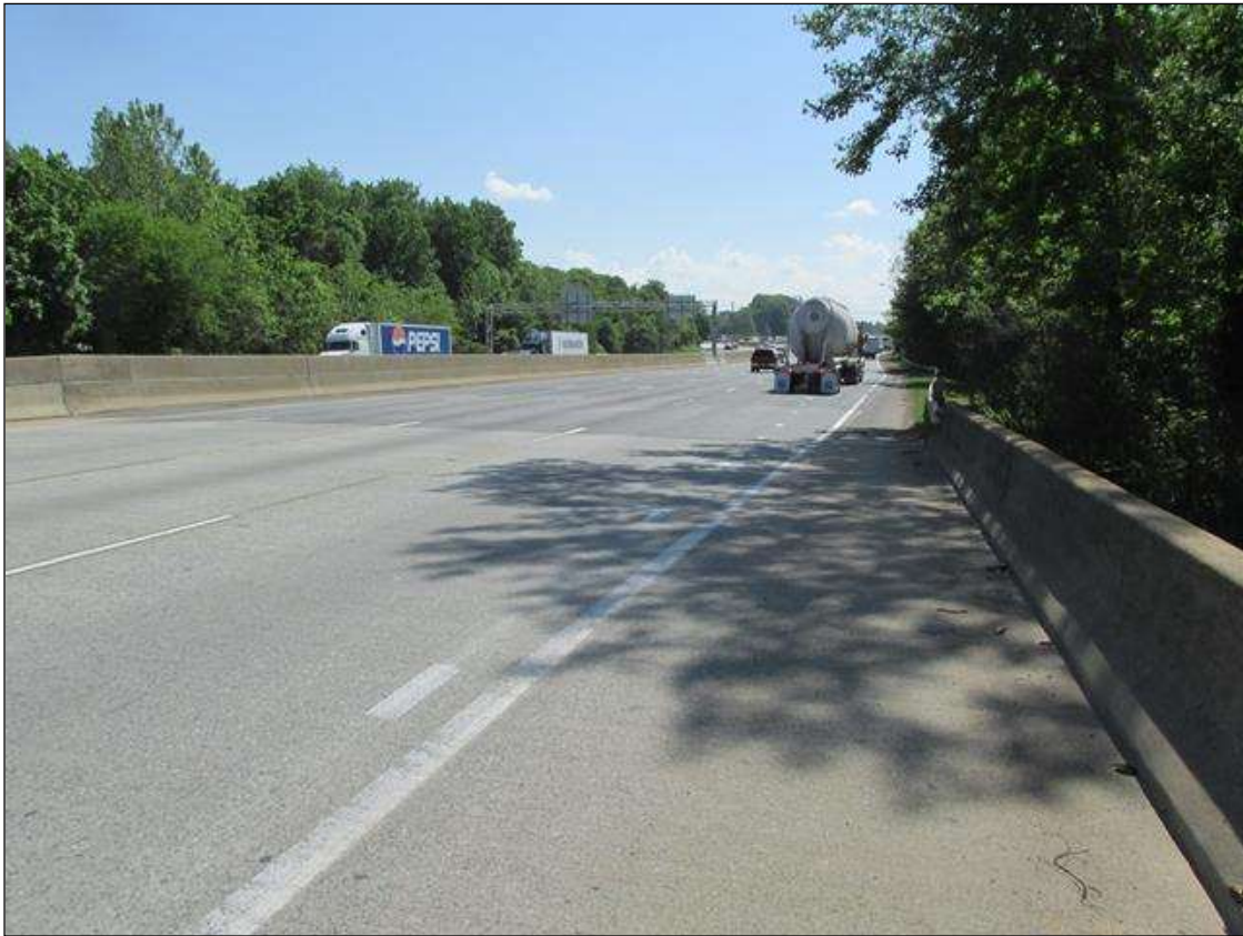
GUARDRAIL LOOKING NORTH, -L- RT
