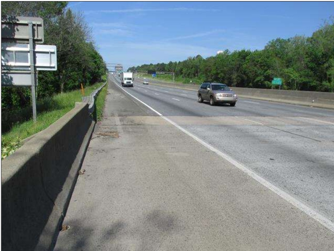
GUARDRAIL LOOKING SOUTH, -L- RT
