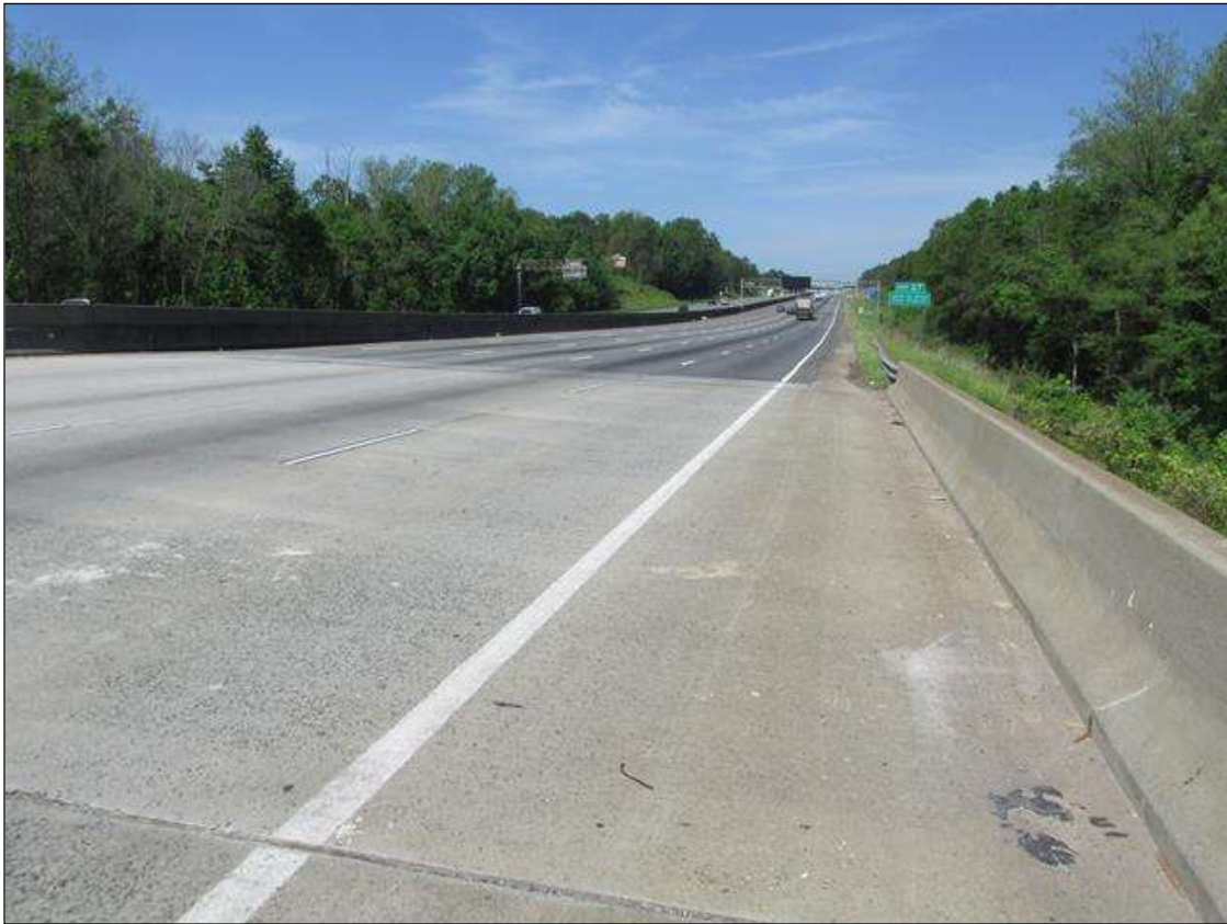
GUARDRAIL LOOKING SOUTH, -L- LT
