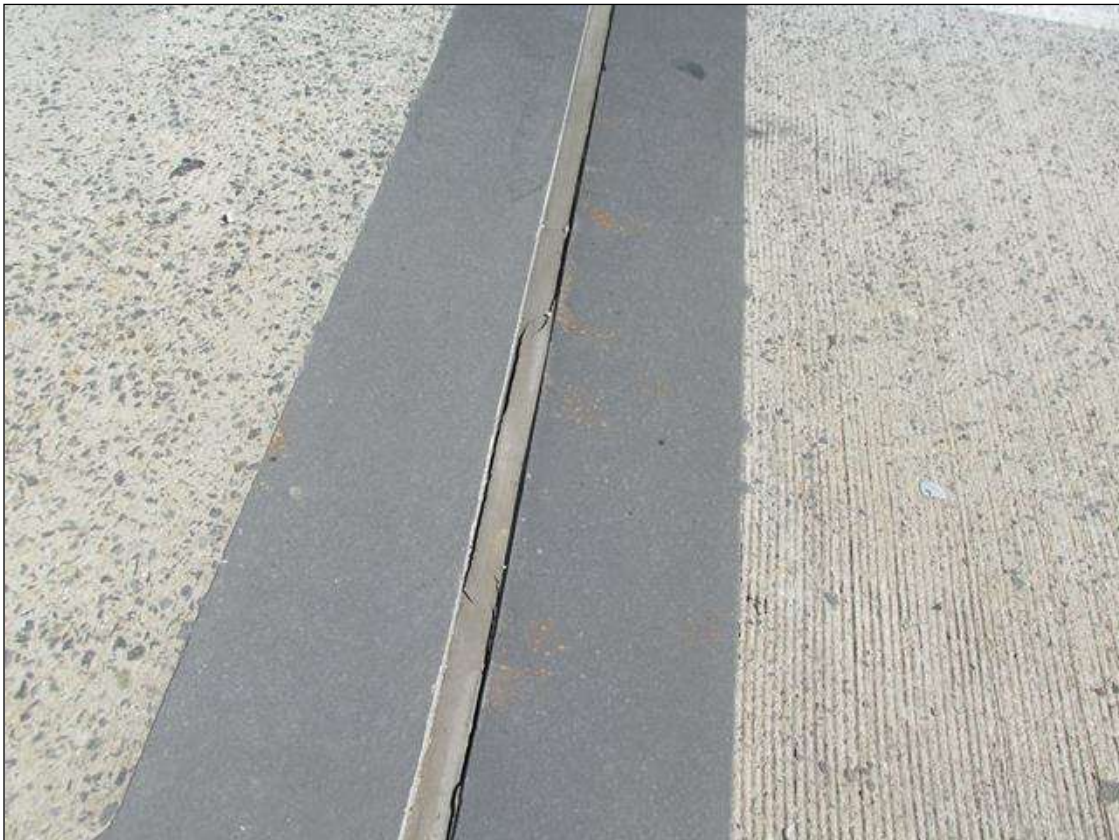
COMPRESSION SEAL AT BENT 9 CRACKED AND OXIDIZED, LEAKING, FULL WIDTH, -L- RT
