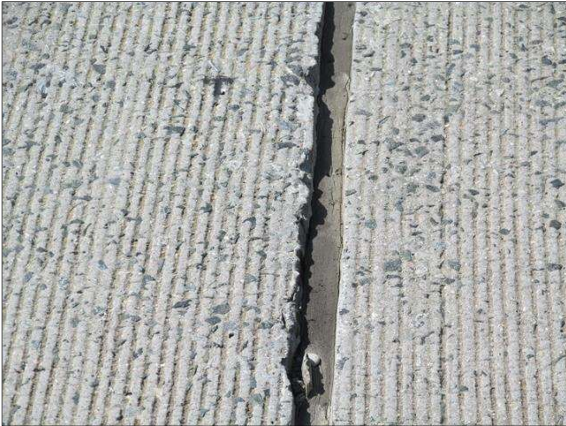
JOINT SEALS OXIDIZED AND SEPARATING ALLOWING LEAKAGE AT BENTS 1-4, & 10, FULL WIDTH, -L- RT AND -L-LT
