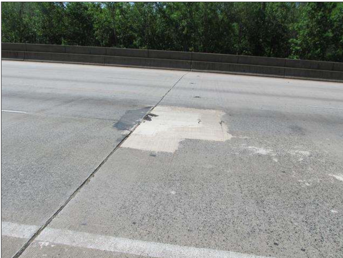
TEMP REPAIR TO DECK IS CRACKED AND POPPING OUT AT BENT 1, -L- LT, APPROX 60SF.
