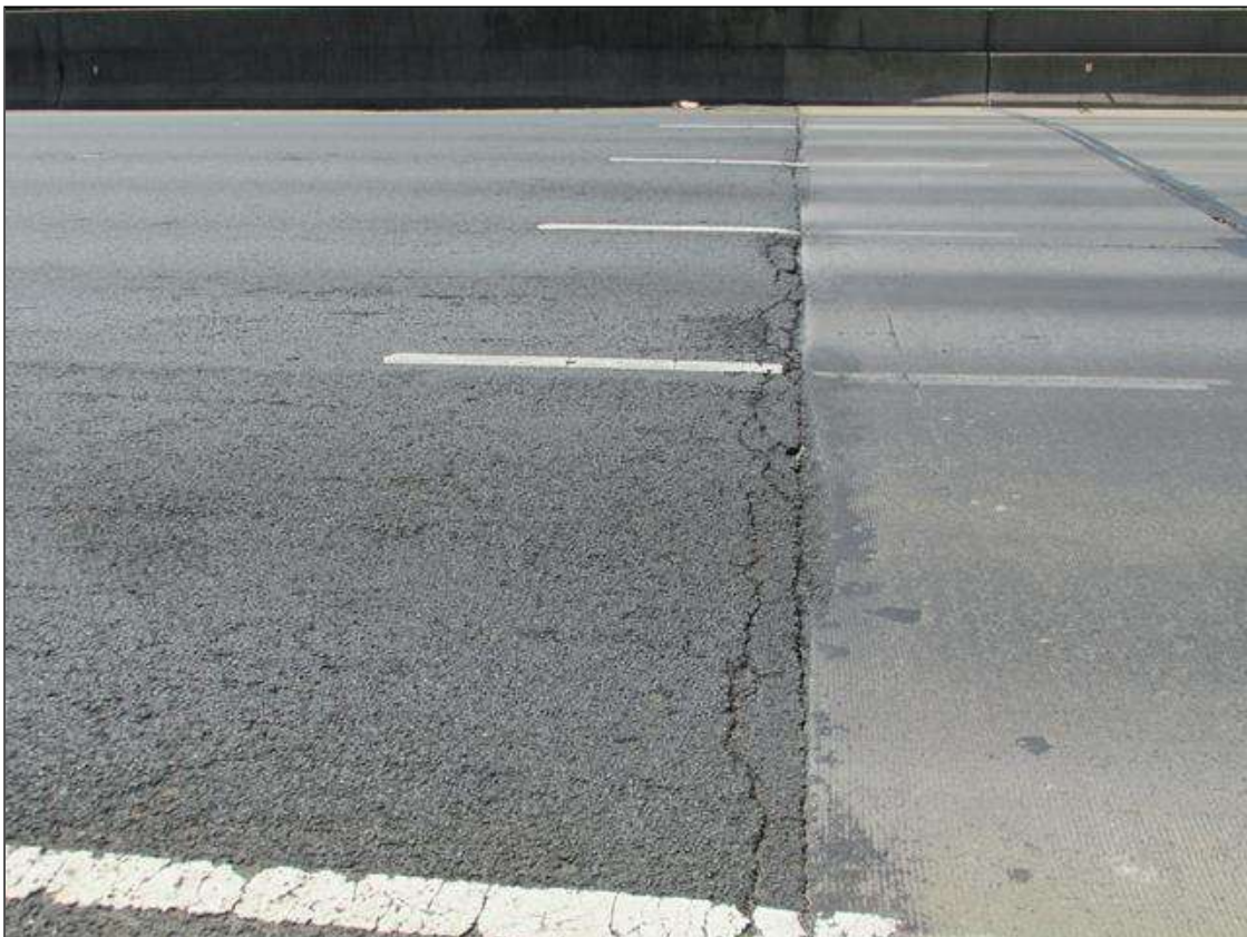
NORTH APPROACH ROADWAY CRACKED AND LOOSE ALONG APPROACH SLAB, -L- LT, APPROX 5SY
