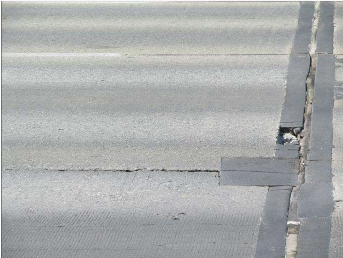
TEMP REPAIRS TO DECK AND APPROACH SLAB AT NORTH APPROACH, -L- LT. REPAIRS ARE CRACKED AND POPPING OUT. APPROX 10SF.
