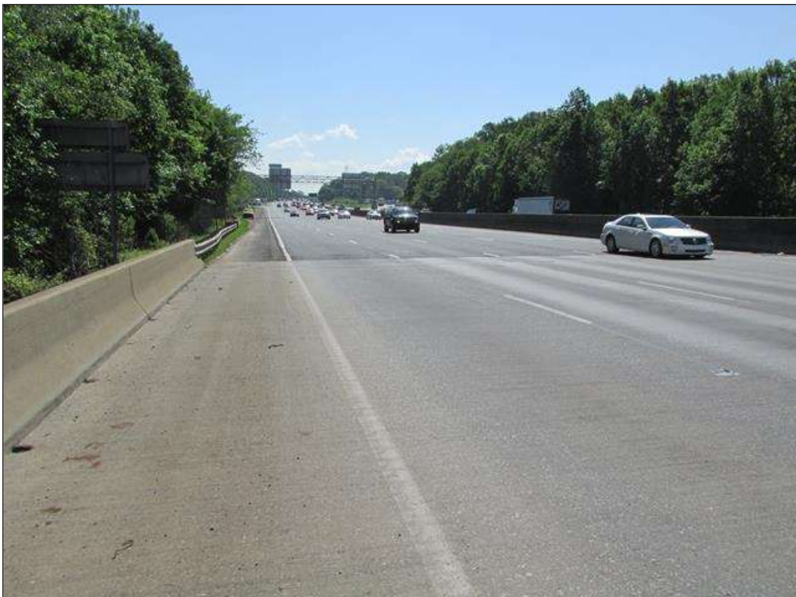
GUARDRAIL LOOKING NORTH, -L- LT
