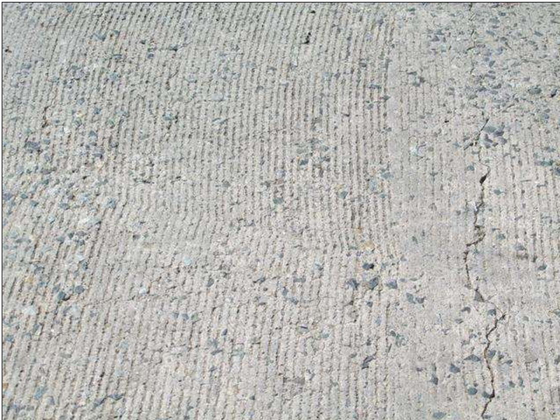
SCATTERED HL CRACKING THROUGHOUT TOP OF RC DECK
